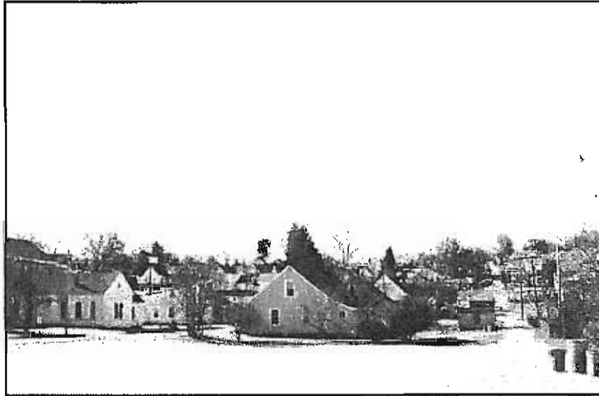
Lockhart Mill Village, looking north from the Mill Site.
