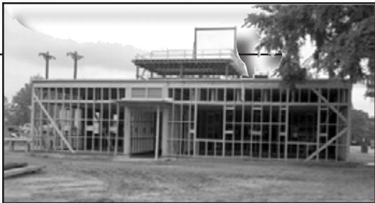
*View of Joist Construction of Building 679 (CMX), 1951 (SRS Neagative # 6-121).*
