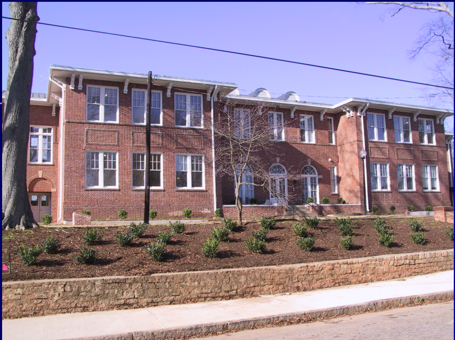
Kennedy Street School Anderson, South Carolina
