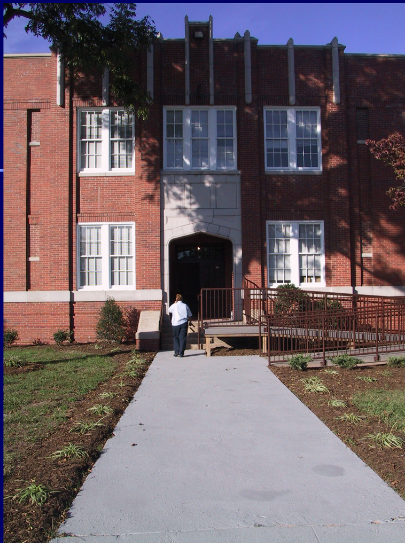
Central School Bessemer City, NC
